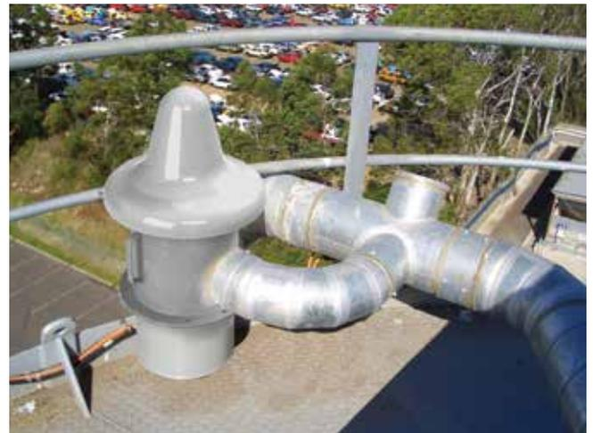
VHS Pressure Relief Valve releasing excess pressure
